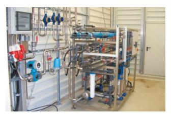
With the dual level reverse osmosis system, both an-organic as well as organic highly contaminated waste water can be treated.
